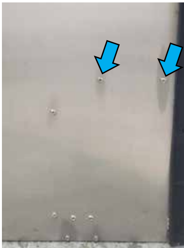
Step 14: Rivet the new condensate evaporator assembly in place.
