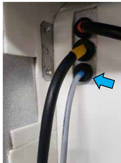
Step 15: Tie the wire left from old condensate evaporator in order to pull the cable of the new condensate evaporator. Use grommet removed from the old power connector and press it into place.
