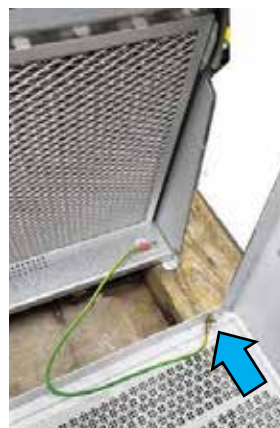
Step 22: Install cover back, connect ground wire before positioning cover.
