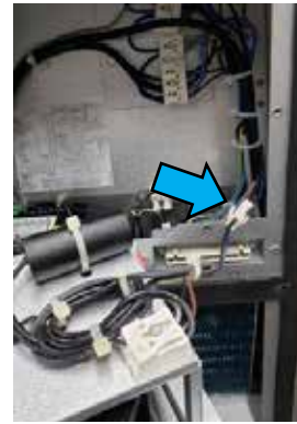
Step 26: Connect internal fan assembly power connector.
