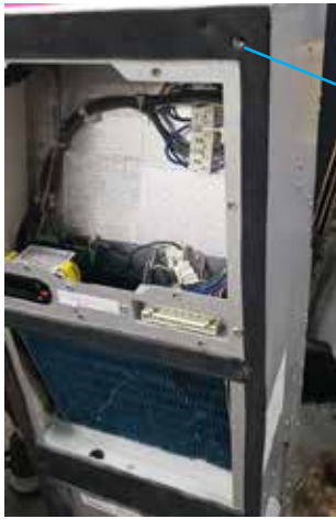
Step 5: Locate power connector for the heater.
