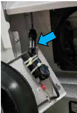
Step 24: Reconnect the ambient fan assembly to connector.
