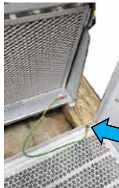
Step 29: Install cover back into place, connect ground wire before positioning cover.
