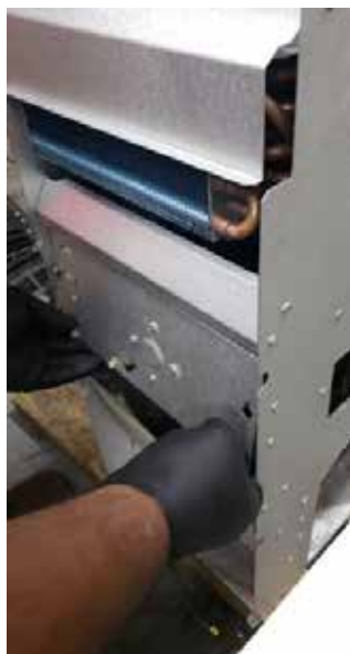
Step 9: Slide assembly up and remove assembly.
